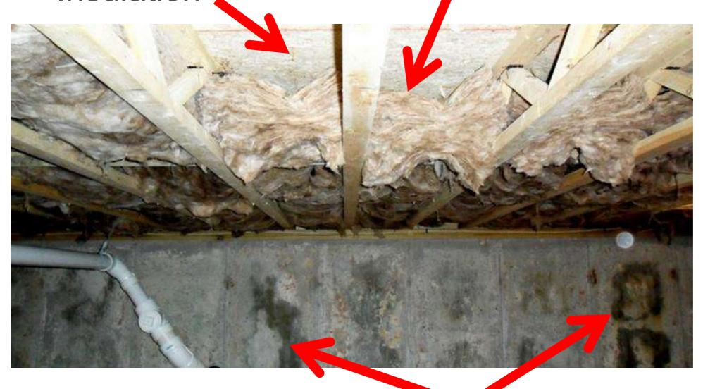
Evidence of bulk moisture and mold
