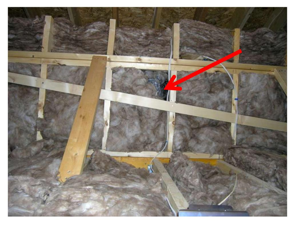
Insulation removed from Kraft facing
